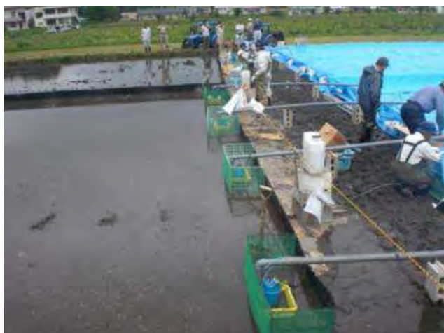
FIG. D.4. Draining suspended soil from paddies in Japan as a remediation option (courtesy of MAFF-NARO).
