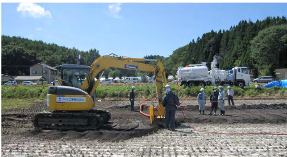
FIG. D.3. Testing topsoil removal after using a soil hardener (Courtesy of Ministry of Agriculture, Forestry and Fisheries (MAFF) / Japan Atomic Energy Agency (JAEA) / National Agriculture and Food Research Organization (NARO), Japan).
